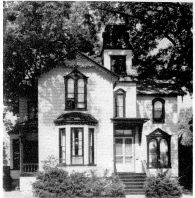
This house at 10330 South Seeley Avenue was built in the 1870s by the Chambers family. Its L-shaped plan, the tall tower, smooth wall surfaces, and decorative exterior woodwork are characteristic of Italianate architecture.
